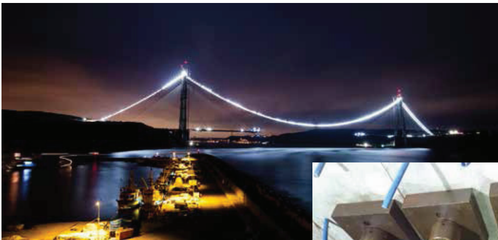
Yavuz Sultan Selim Bridge (aka Third Bosphorus Bridge) Designer Hyundai & SK Engineering JV Installation and Stressing by Intekno
