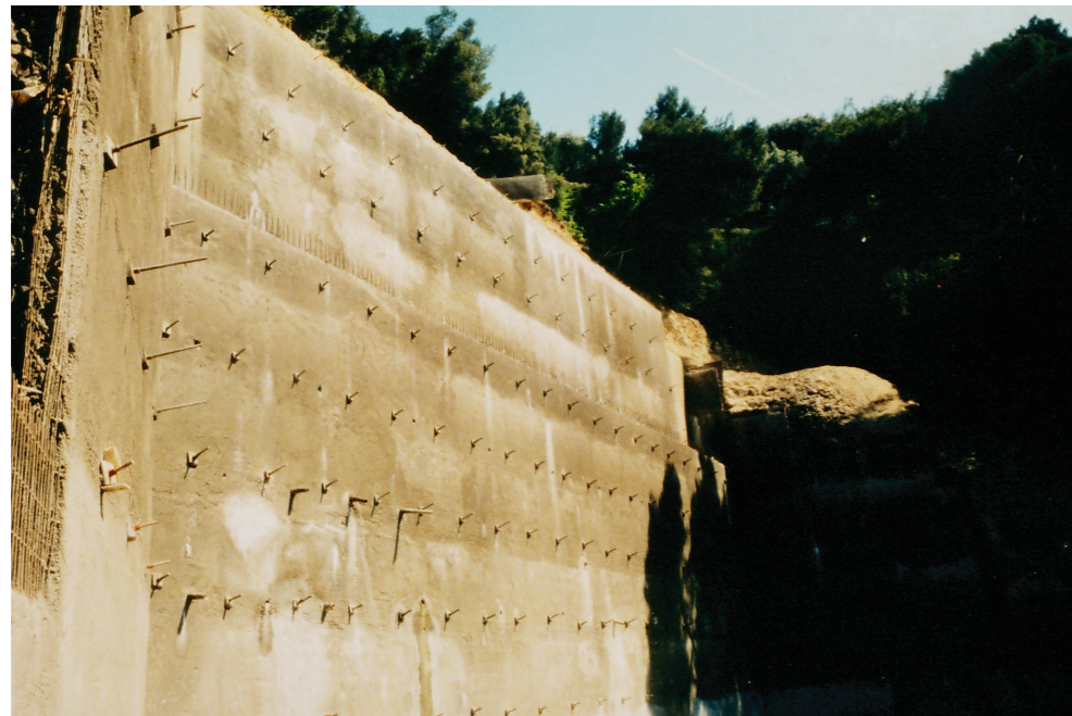
Eugene Corniche Retaining Wall
