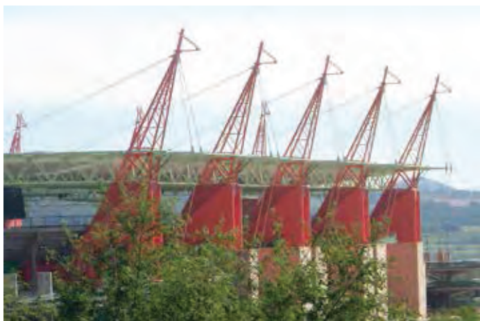
Mbombela Stadium, Nelspruit South Africa Client - Mbombela Local Municipality Structural Engineer - Mott MacDonald
